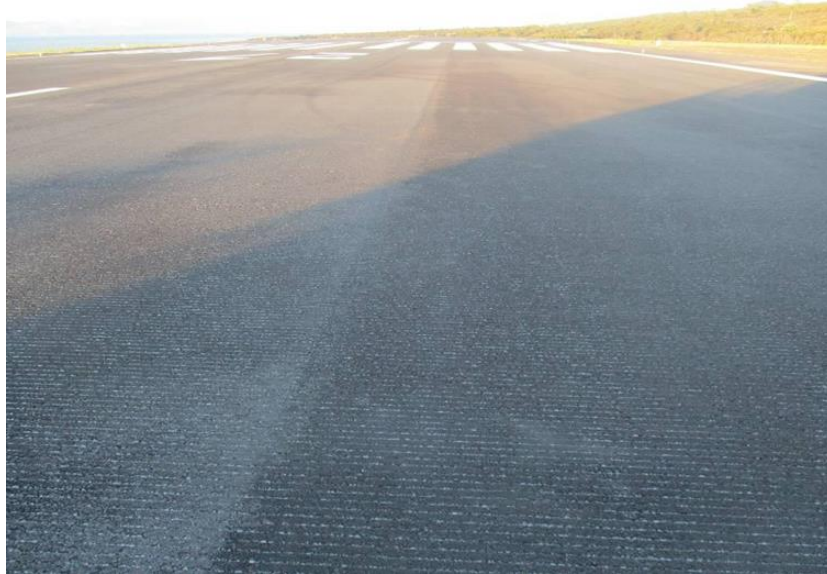
Figure 15. 20 Grooving in Pico runway: detail.
